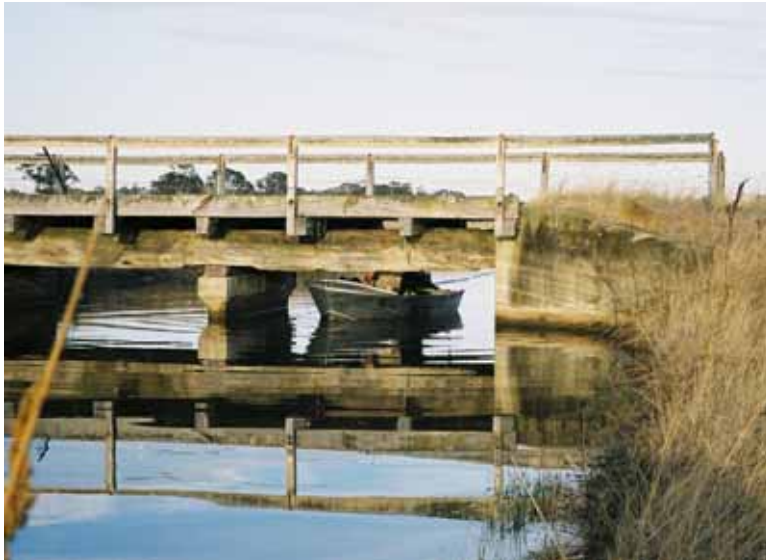
Figure A2-11 Passing under a typical bridge while towing a geo-electric array.
