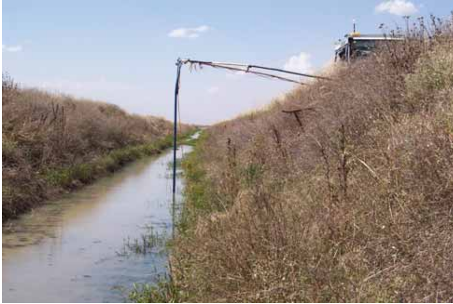
Figure A2-4 The 4.5m boom towing an array along a drain. Note that the boom reach has been exhausted and that a 6 metre boom would be more appropriate at this location.
